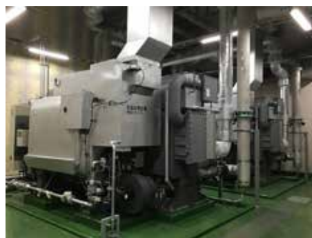
Replaced hot / cold water generators at Fujiyama Works
